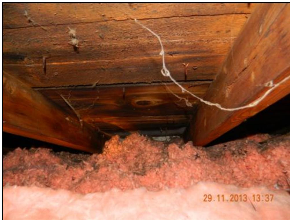
1.5 Picture 1 ATTIC VIEW
