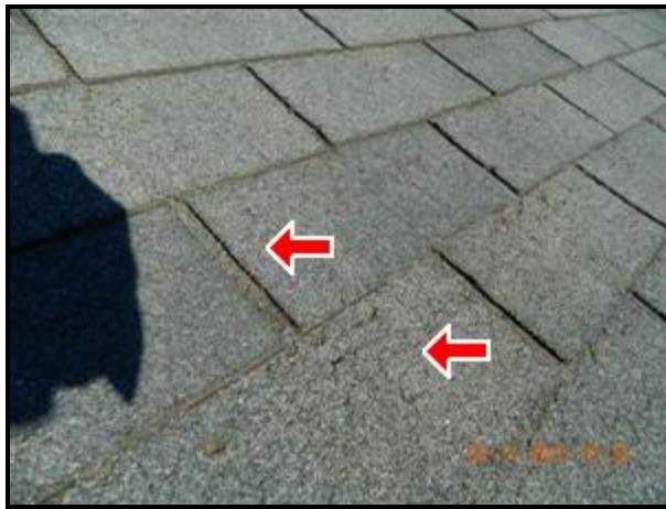
3.0 Picture 1 ROOF SHINGLE VIEW
