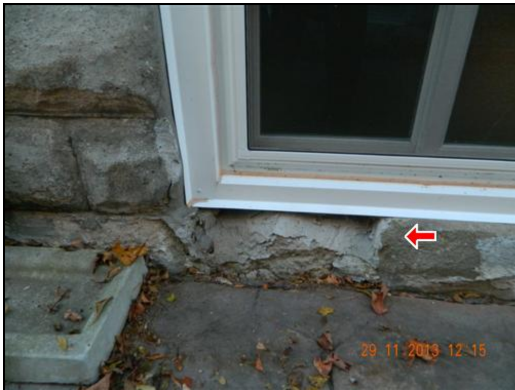
1.0 Picture 1 NORTH SIDE
