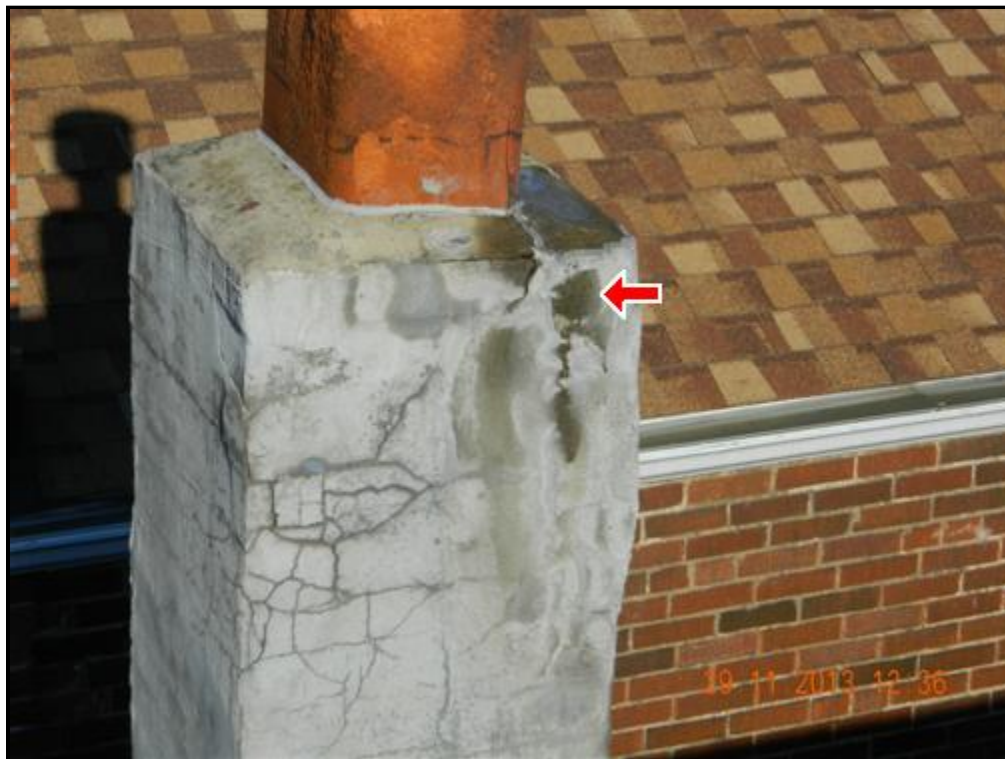
3.2 Picture 1 CHIMMEY VIEW
